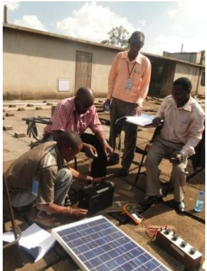
Participants installing a solar system
